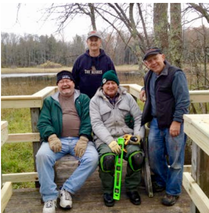
Observation Deck Repair
